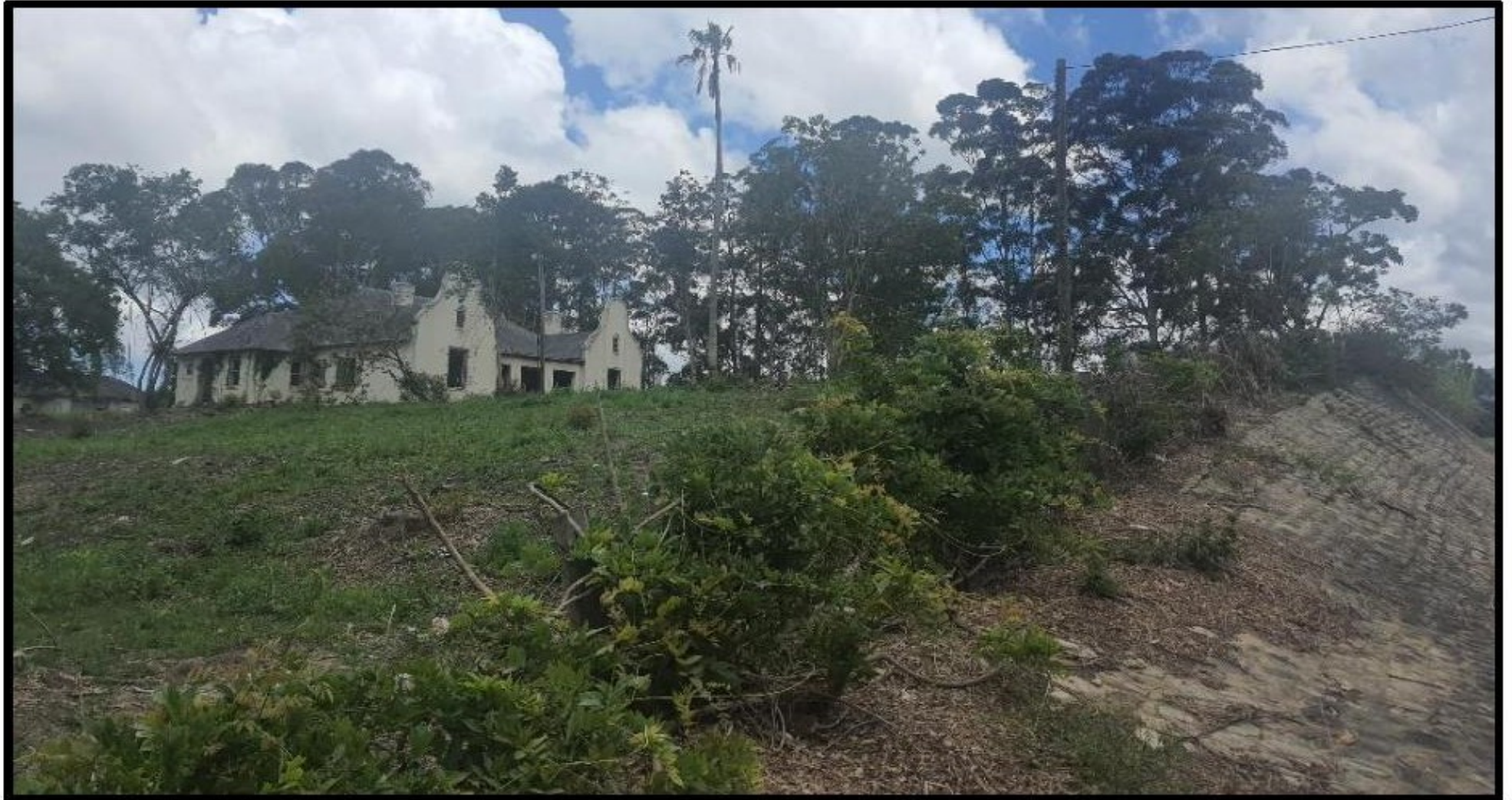
Figure 3a: Site Photos
