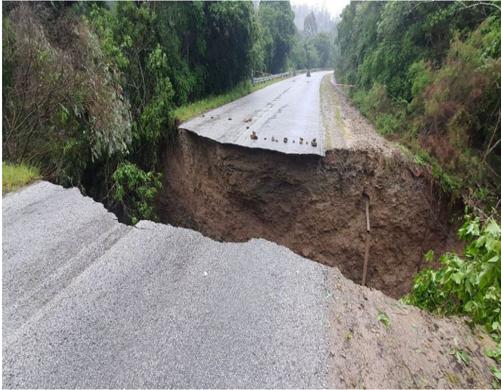
Figure 1: Slip failure, Armco washed away
